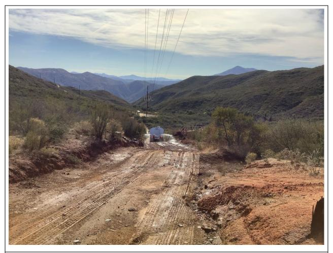
**Photo 1:** During access road maintenance along TL 6923, a water tender was observed applying water to the road to minimize dust emissions in accordance with APM AIR-02.
