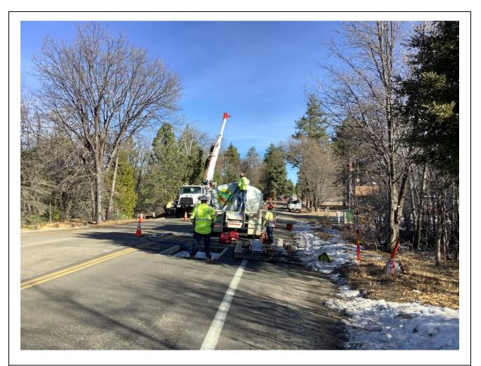
**Photo 6:** During dewatering activities on C 440, groundwater was pumped into a truck-mounted storage tank and transported to an authorized discharge location in accordance with APM HYD-08.
